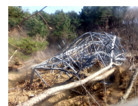
Loss of off-site power due to destruction of transmission line
